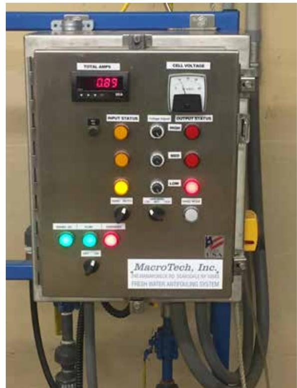
Copper Ion Generator Technology uses electrolytically produced ionic copper to control veliger settlement.
